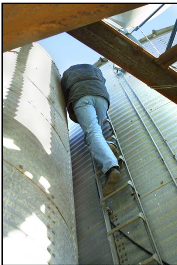
Photo 3 – View from the ground looking up the old grain bin ladder.
